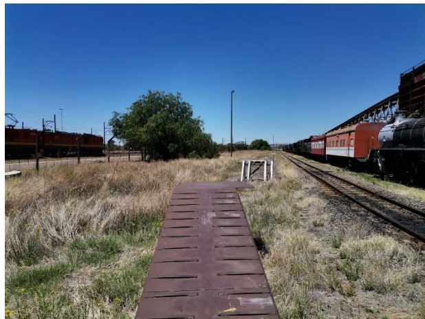
8. Existing railway structure on site
